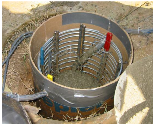
Figure 4.2 Arrangement of reinforcing bars and vinyl tubes
